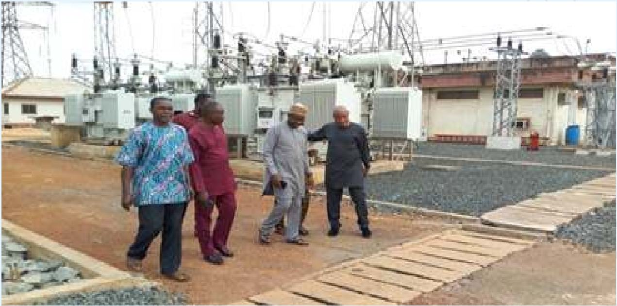
MD and Head TCN Inspecting 2X60MVA Installed by MBH at New Haven 330kV S/S
