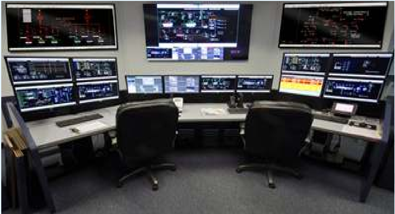
(SCADA Control Room)
